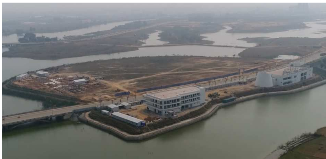
Construction in Hoa Lac High-Tech Park
